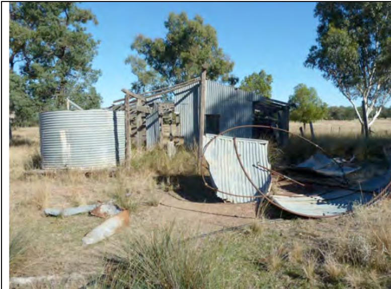
Figure 17 Site VH6, Spray Dip and Shed. Spray dip equipment in foreground.
