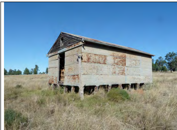
Figure 18 Site VH7, Shed.
