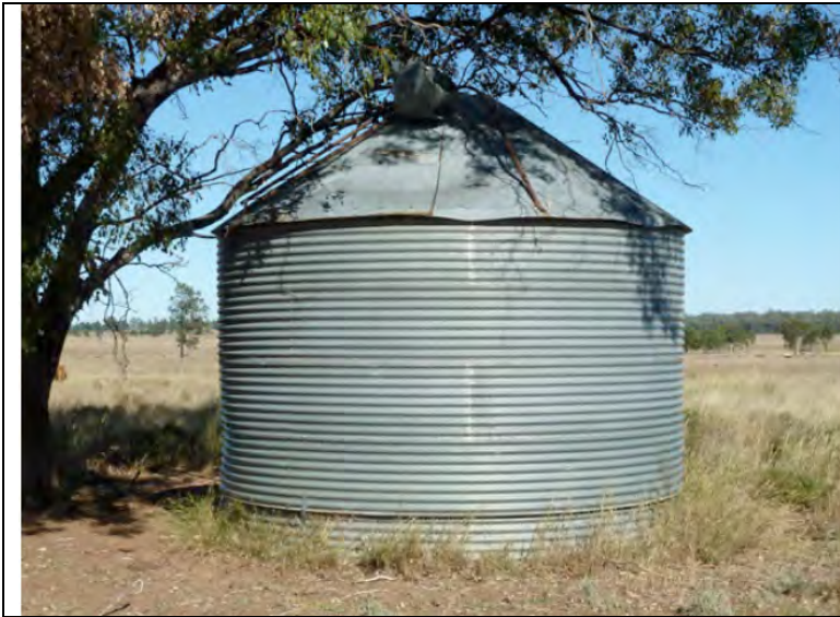
Figure 24 Site VH8, Wilga Homestead Complex. Silo.
