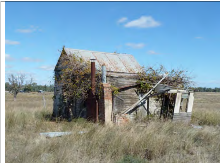
Figure 34 Site VH11, Cottage and Shed. Cottage.
