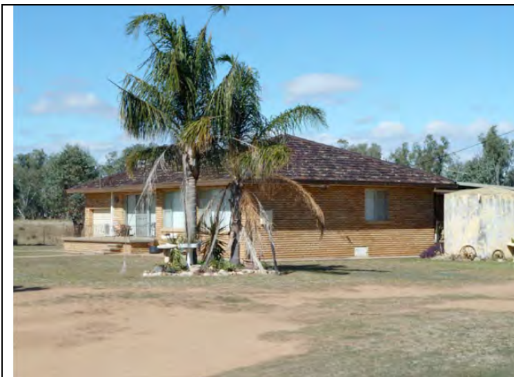
Figure 40 Site VH12, Broadwater Homestead Complex. Brick cottage.
