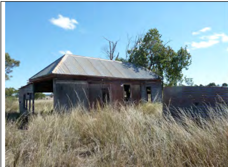
Figure 30 Site VH10, Cottage. View from south-east
