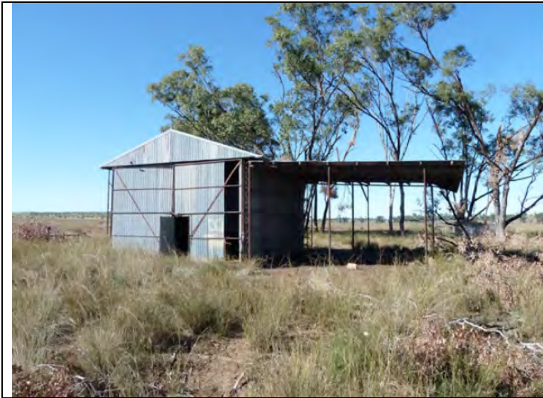
Figure 21 Site VH8, Wilga Homestead Complex. Shed 1. Steel-framed CGI clad shed with skillion shelter for truck.
