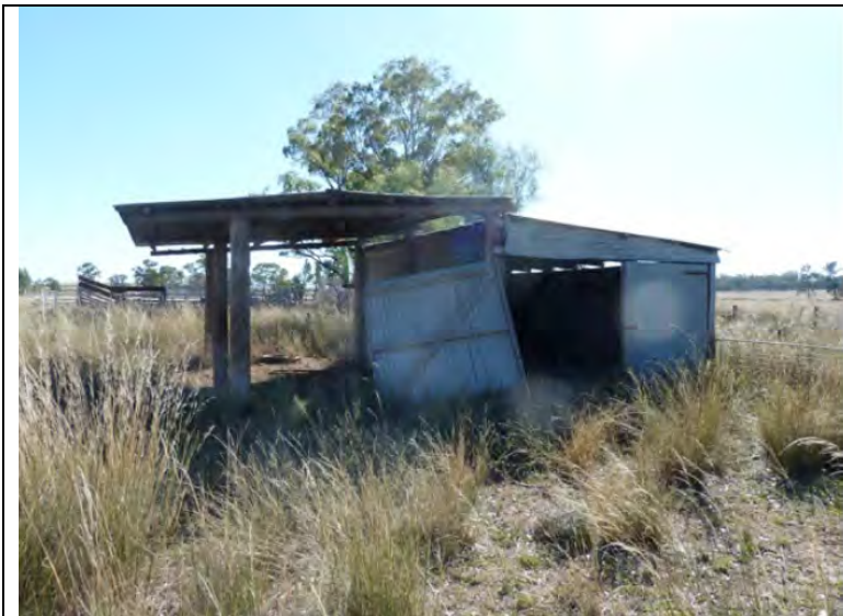
Figure 22 Site VH8, Wilga Homestead Complex. Shed 2. Workshed and skillion.
