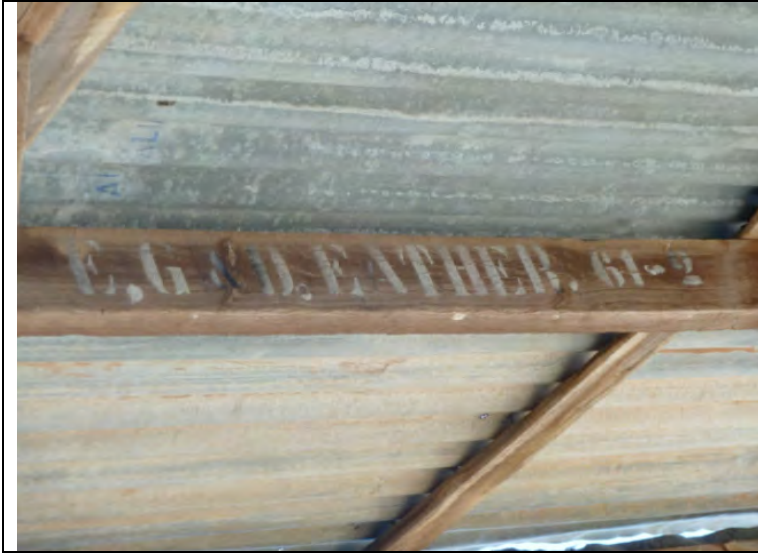
Figure 29 Site VH9, Shearing Shed. Stencil on roof frame.
