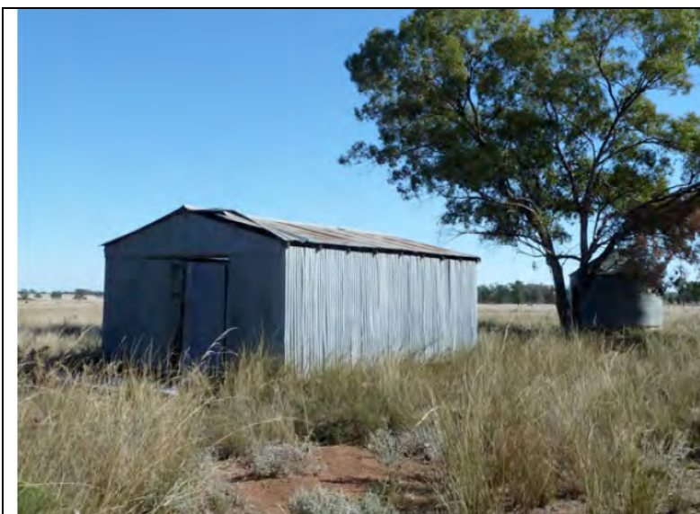
Figure 23 Site VH8, Wilga Homestead Complex. Shed 3.
