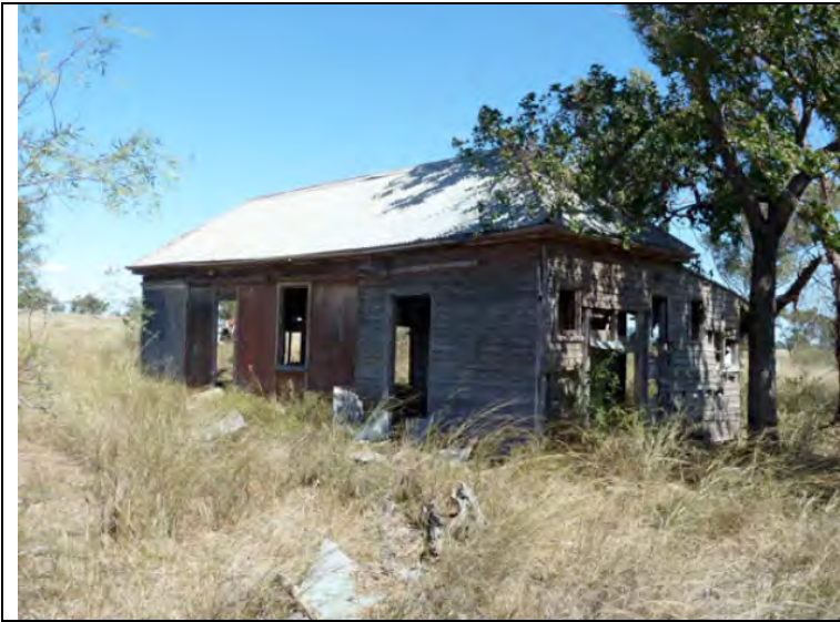
Figure 31 Site VH10, Cottage. View from north-east.
